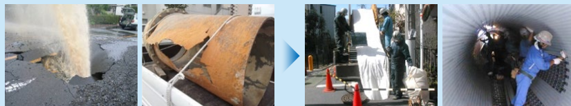
Increasing number of aging pipelines
