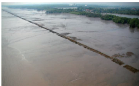
図-1 Geo-Tube 製離岸堤 (Marine Department 提供)
